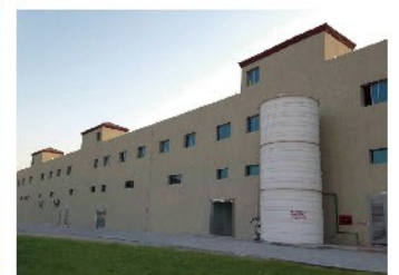
Randhal Project-United Arab Emirates
